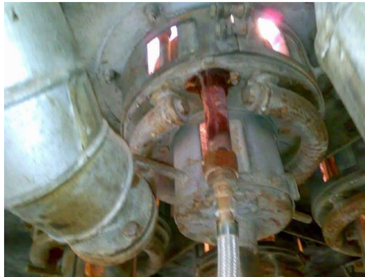
Fig.e: Which shows low NOx burner with two air boxes
